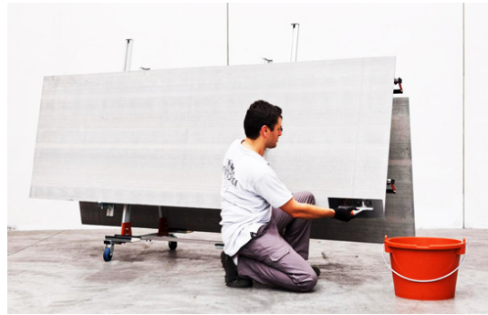
Back-buttering on transport cart
